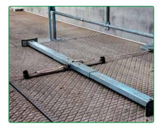
The rope scraper installations always contain 2 drive units. When one of the drive units is winding the rope, the other one will release the rope at the same time. Therefor it is not necessary to tension the system. Rope scraper systems are animal friendly and require little maintenance and service.
